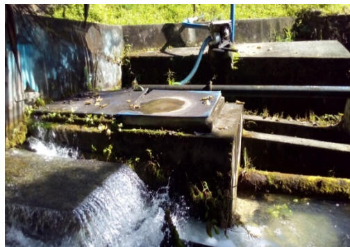
Figure 2. Mangkio water spring building.
