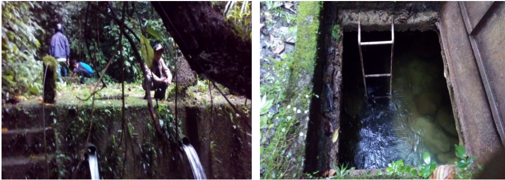
Figure 1. Keles water spring building.
